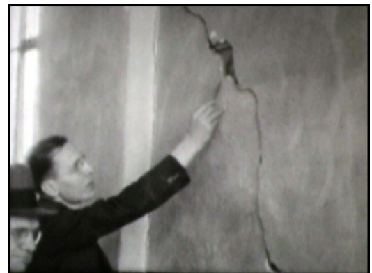
Superintendent George Rilling points out one of the cracks in the school gymnasium caused by the March 2nd earthquake.
